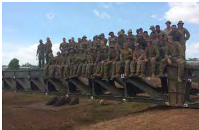
3 Tp constructing an MGB
