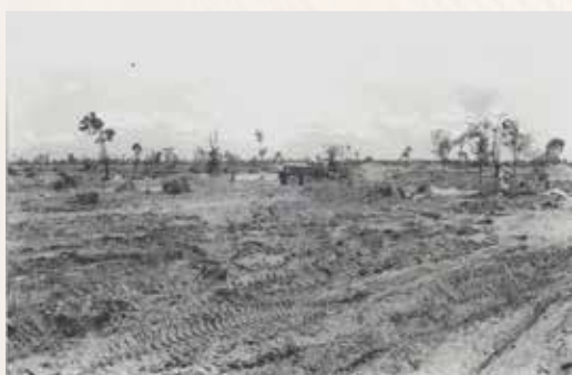
Clearing and construction at Coral
